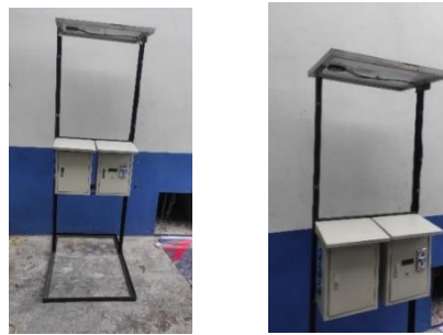
Fig 6. The SPKLU design is coin-operated
