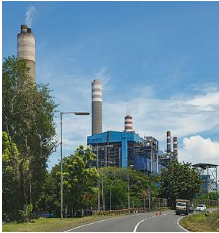
Fig. 4. Steam power plant at PT POMI Paiton
