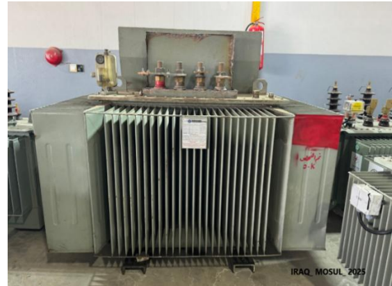
Fig. 2. Shows a real model of the exterior of a 1000 kVA transformer at the maintenance center in Mosul, Iraq
