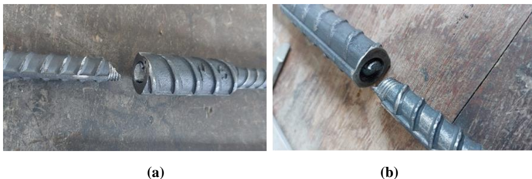
Figure 11. Fracture necking failure in D16 (a) and D13 (b) reinforcement bars
