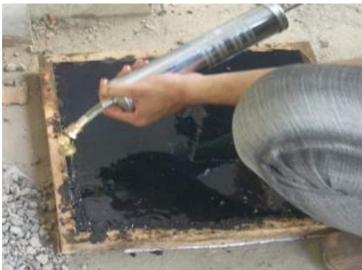
FIGURE 4. The resin is sprayed on the top of HRS with thickness 2/3 ALD
